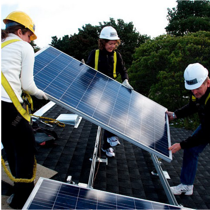
Wells Fargo team members install solar on a home in California — Courtesy of Grid Alternatives
