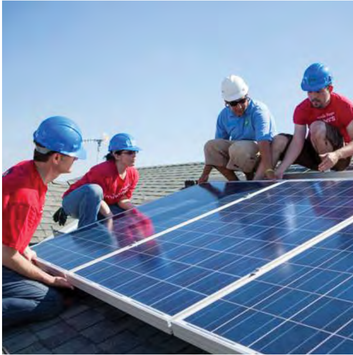
Wells Fargo team members installing solar panels at a home in Fresno, CA, with Grid Alternatives.
